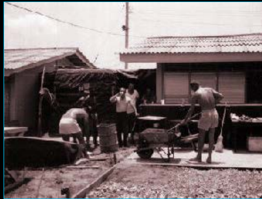
5) NCOs working hard building a patio.
