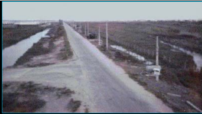
4) The perimeter road from tower.
