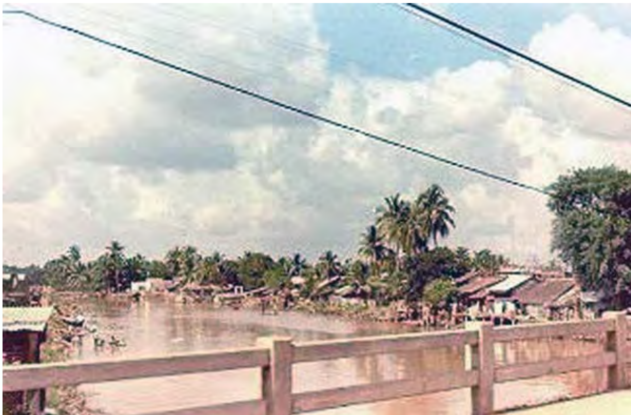
46) Bridge to Can Tho.
