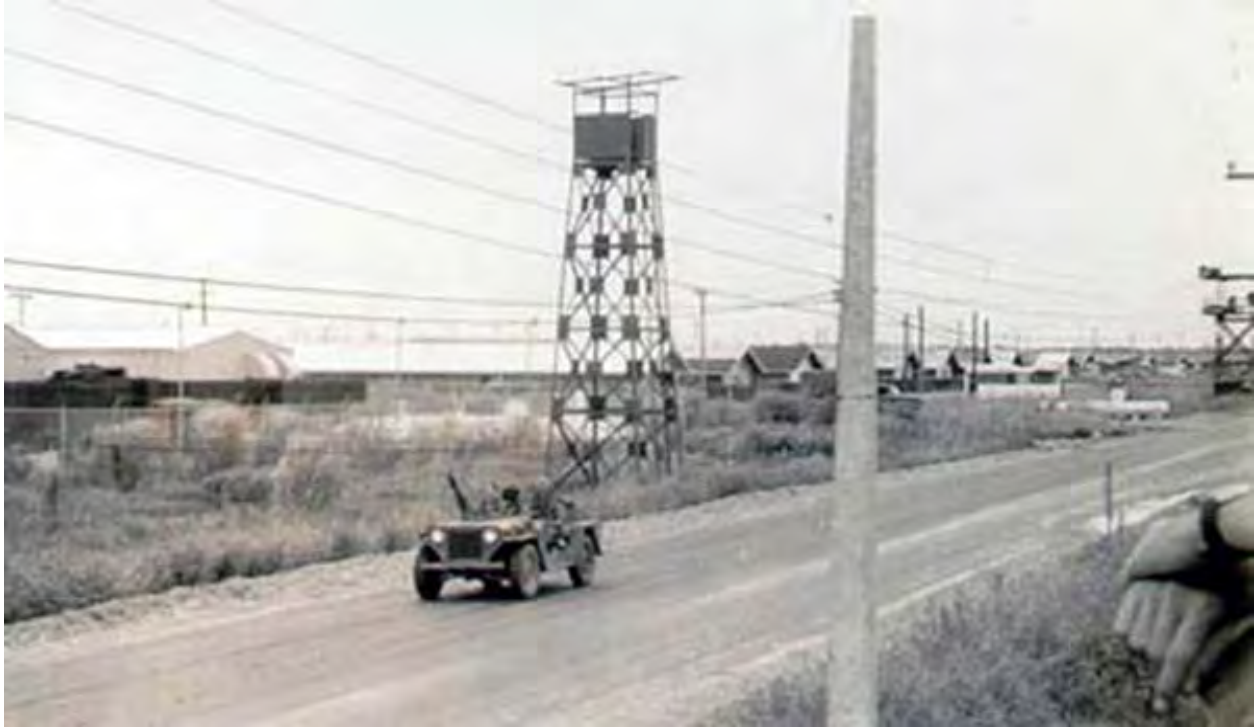
18) Perimeter Tower and Pole.
