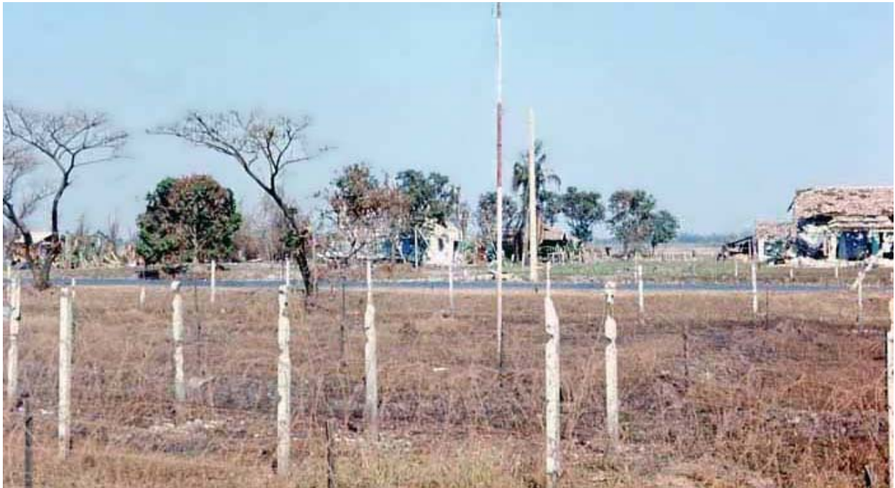
Tan Son Nhut AB, 377th SPS, perimeter-fence after TET 1968 attack. MSgt Summerfield: 09
