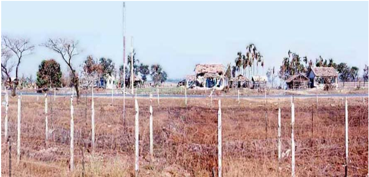
Tan Son Nhut AB, 377th SPS, perimeter-fence after TET 1968 attack. MSgt Summerfield: 08
