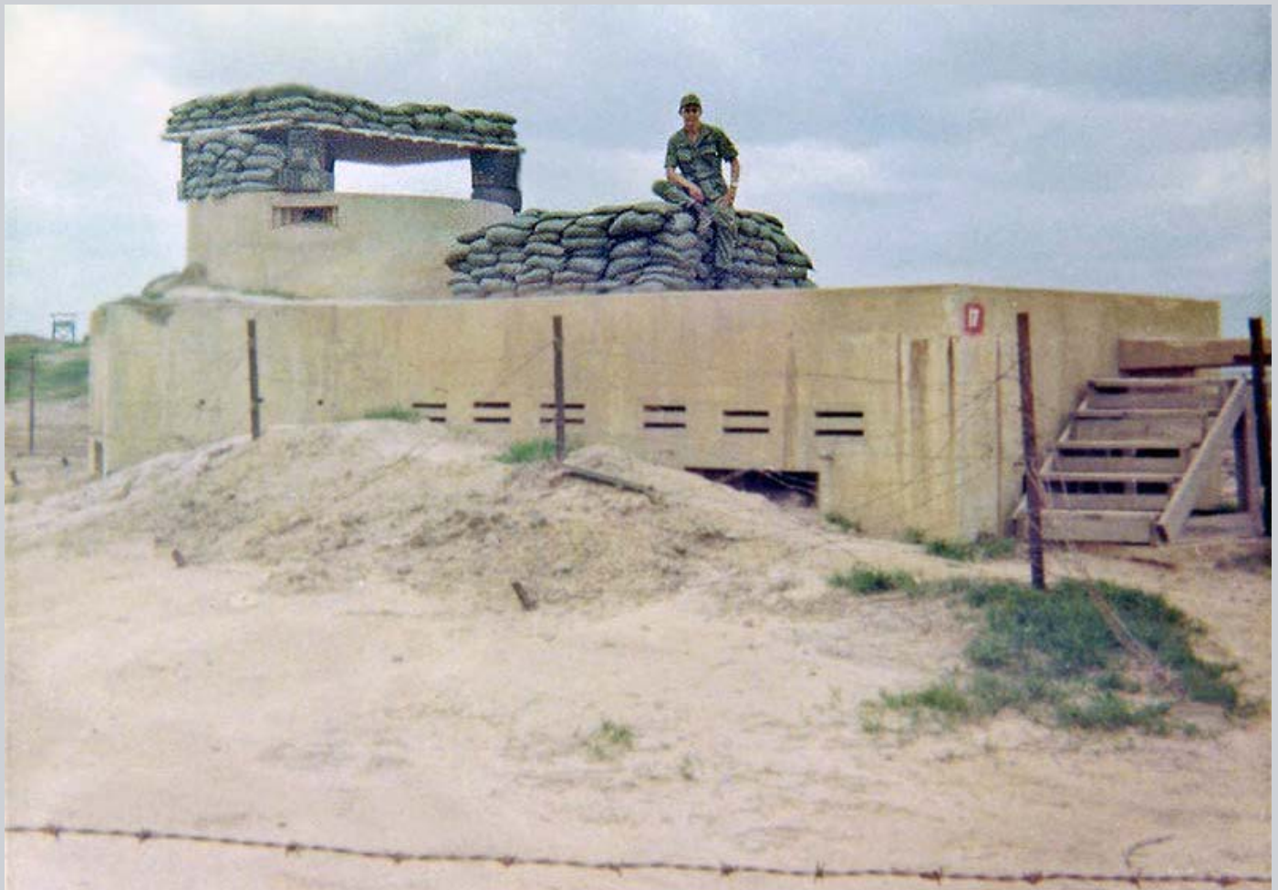
8. Biên Hòa AB, Bunker-17. Tower (center-left) 1966-1967. Photo by Ernest Govea, BH, 3rd SPS, 1966-1967.
