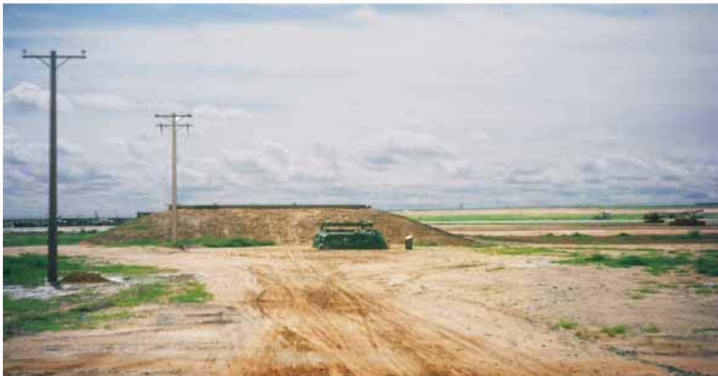
12. Biên Hòa AB, Bunker-1, with a shack next to it, looks like it may be ARVN or VNAF security. Photo by Bob Vitray, LM 590, BH, 3rd SPS, 1967-1969.
