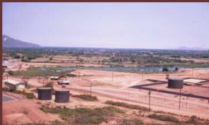
6. Fuel storage are
