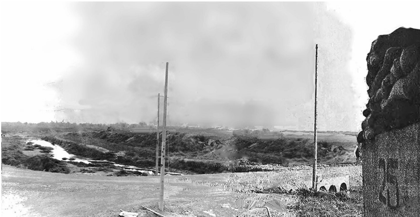
Bunker Hill-10: Perimeter Road. Ditch and culvert under road where VC crossed through.
