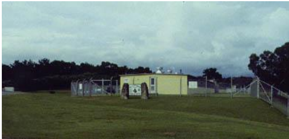
Photo Above: PACAF MWDTC, End of Indoor kennels with kitchen in center. The support building containing two classrooms, administrative office, and the vet clinic is not seen in this photo.
